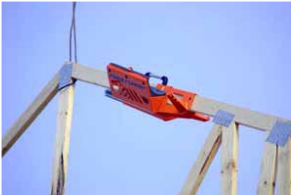
Photo 1. Ridge Runner™ installed on top chord of truss.
