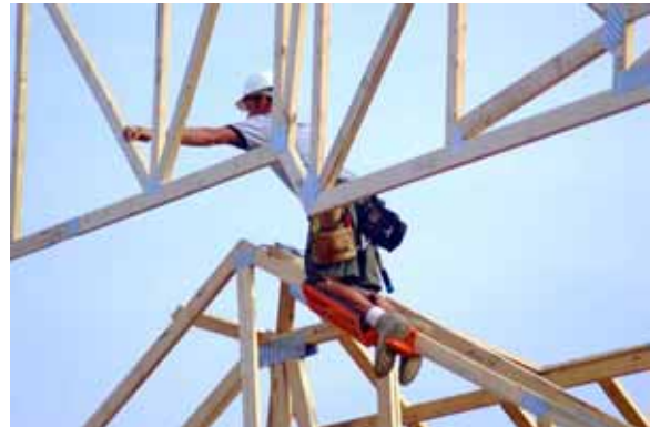
Photo 2. Worker using the Ridge Runner™ to install trusses.
